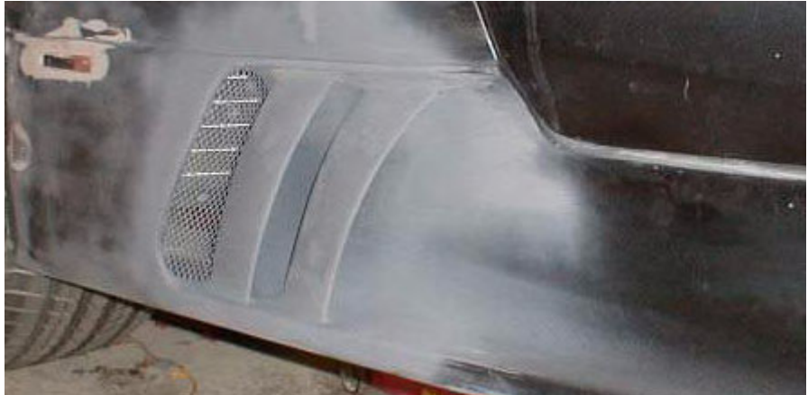
FIGURE 68. Final louver assembly
